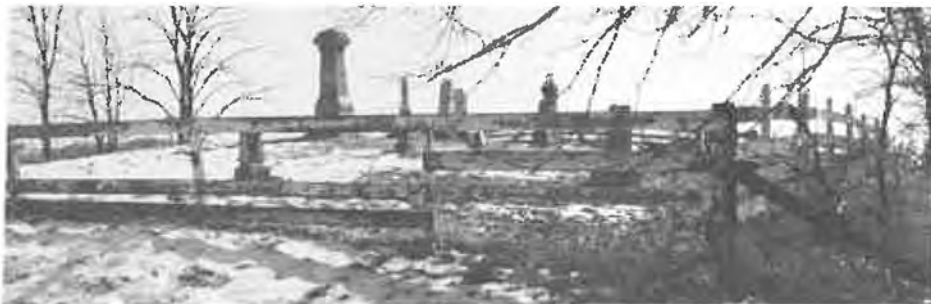
View from north
